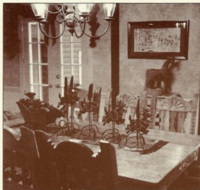
Dining room addition to the one-room schoolhouse done in 1990
