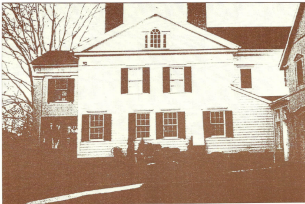
The north face of the original house. The two fireplaces and the placement of windows indicate that the room on the first floor was originally two rooms.
